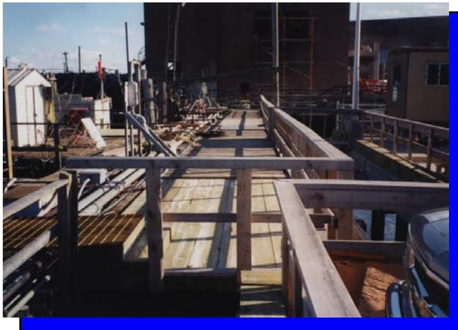
Atlantic Engineering, LLC was summoned for an emergency inspection of the fuel pier. The pier displayed severe deterioration of primary structural members and was exhibiting excessive deflection under ship and barge berth loading. AE performed inspection above and below water with immediate repair recommendations for deteriorated structural elements and design of a temporary fender system. The facility is critical for the operation of the Staten Island Ferry providing refueling for all vessels.
